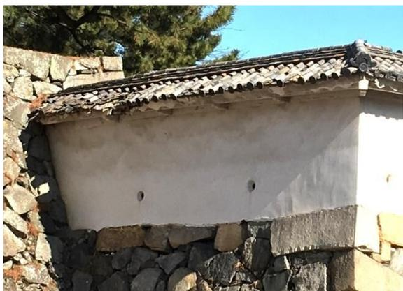
写真 2-9【表二の門附属土塀 (A04')】屋根瓦欠失
